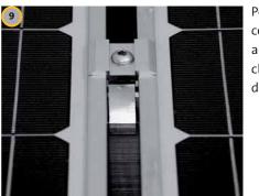
Positioning the second module an adjust the middle clamp to the module frame height
